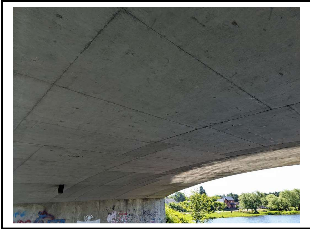
Photo 15 Typical deck soffit
