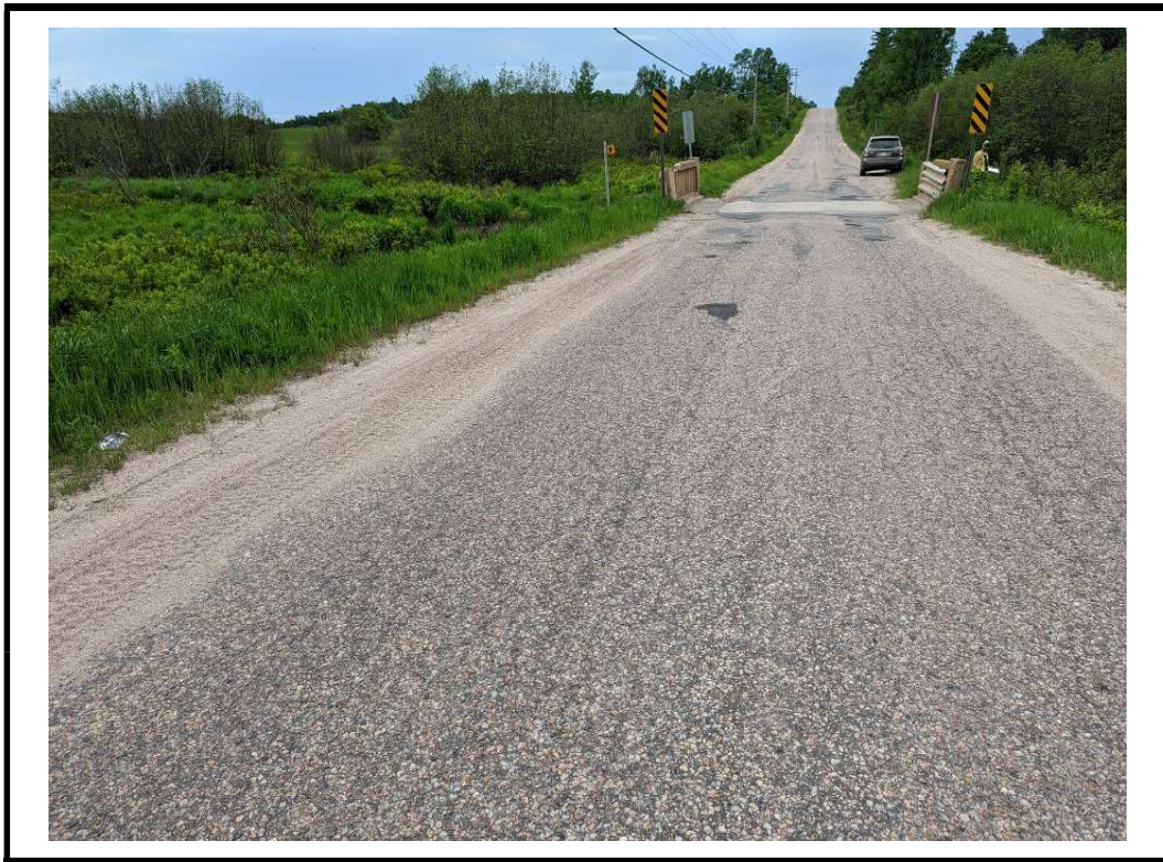
Photo 1 Structure from east approach
