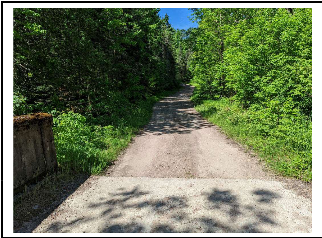
Photo 4 West approach from centre of structure
