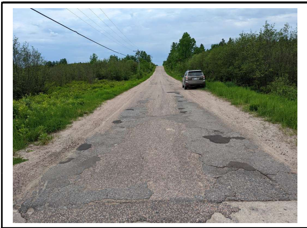
Photo 4 West approach from centre of structure
