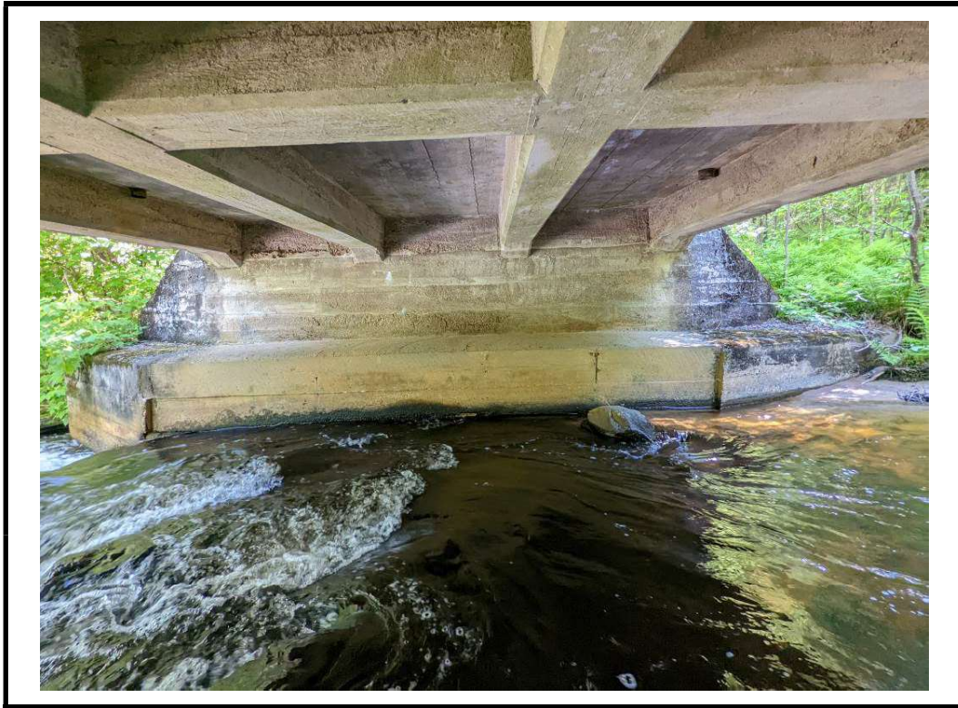
Photo 13 Typical east underside of structure
