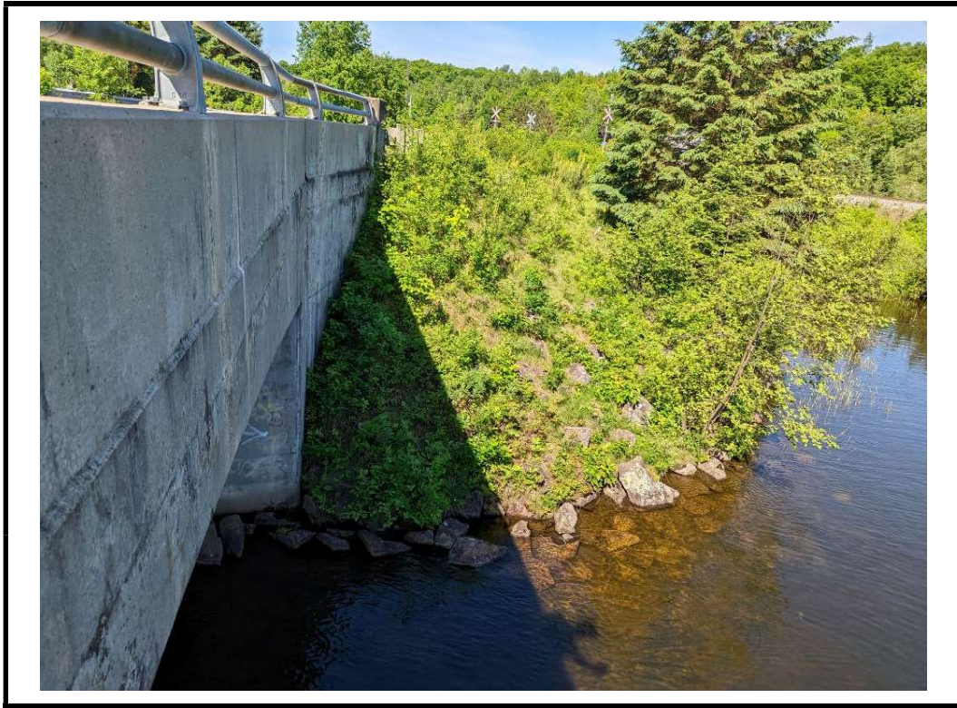
Photo 19 Typical northwest embankment with rock protection at base
