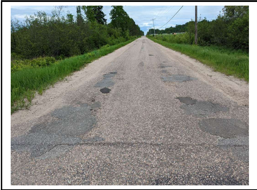
Photo 3 East approach from centre of structure
