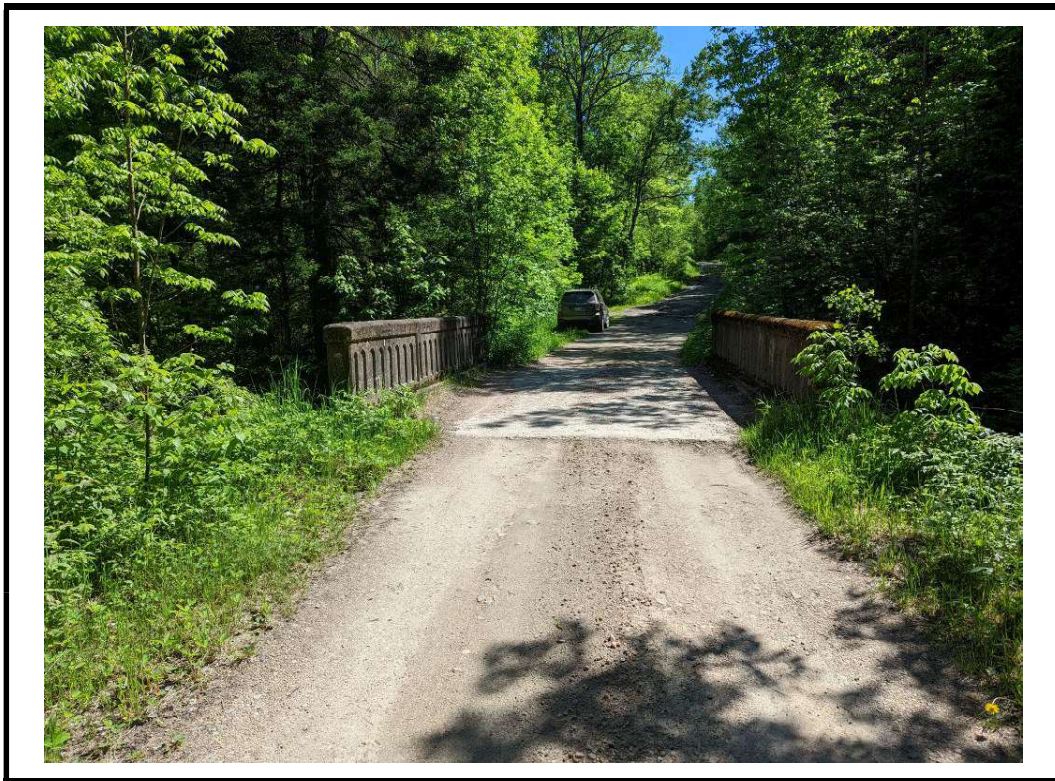
Photo 2 Structure from west approach
